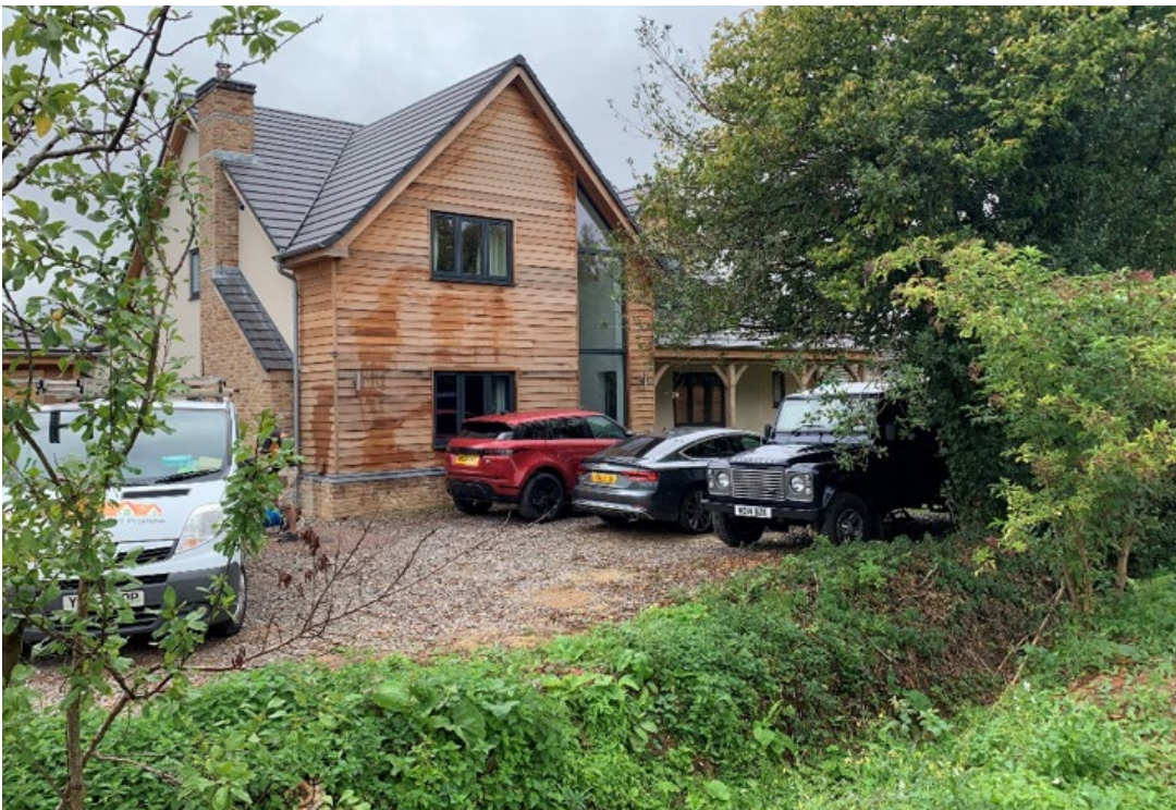
Figure 4: The recent completion of a stunning, substantial, modern 6no. bed dwelling in the village of Rangeworthy (Ref. PT18/5334/F). Materials are a mix of traditional and contemporary; rendered masonry walls with feature cedar cladding to the gables.
