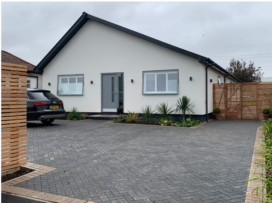
Figure 2: This new single storey dwelling on Hortham Lane, Almondsbury, replaced an existing 3no. bedroom bungalow with a more modern, open plan, family home (Ref. PT18/4878/F). An asymmetric roof modernises this bungalow, as well as the addition of a side dormer window, which increases daylight into the living space. The owners decided to demolish the existing dwelling and build a fit-for-purpose modern, family home.
