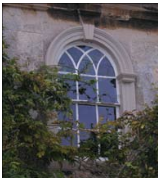
Early nineteenth century plain arched sash window with Gothic style glazing bar decoration.
