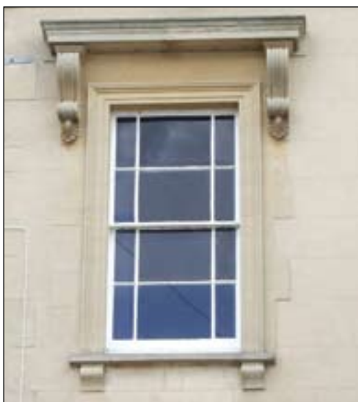
Sash window with marginal glazing and moulded stone surround on corbels, and hoodmould on decorative brackets.
