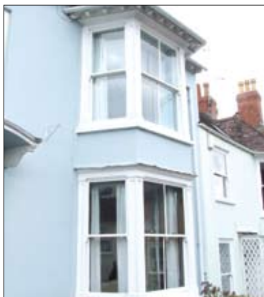
Victorian sashes with large panes and horns.
