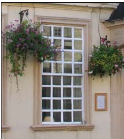
Early sash window with small panes and wide glazing bars
