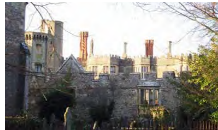
5b Thornbury Castle showing main components of the castle including Tudor chimneys and the wall between the castle and church.
