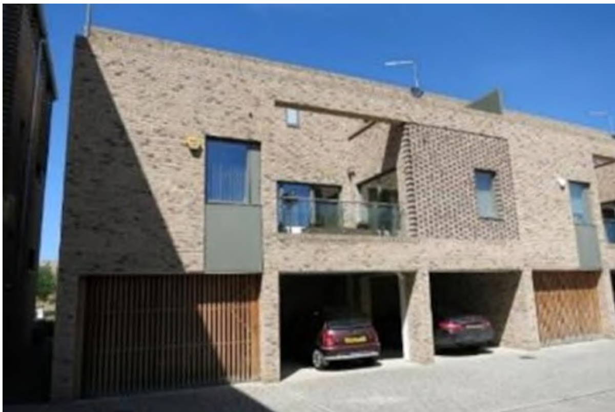
Undercroft and integrated, wide garage parking, Abode, Cambridge.
