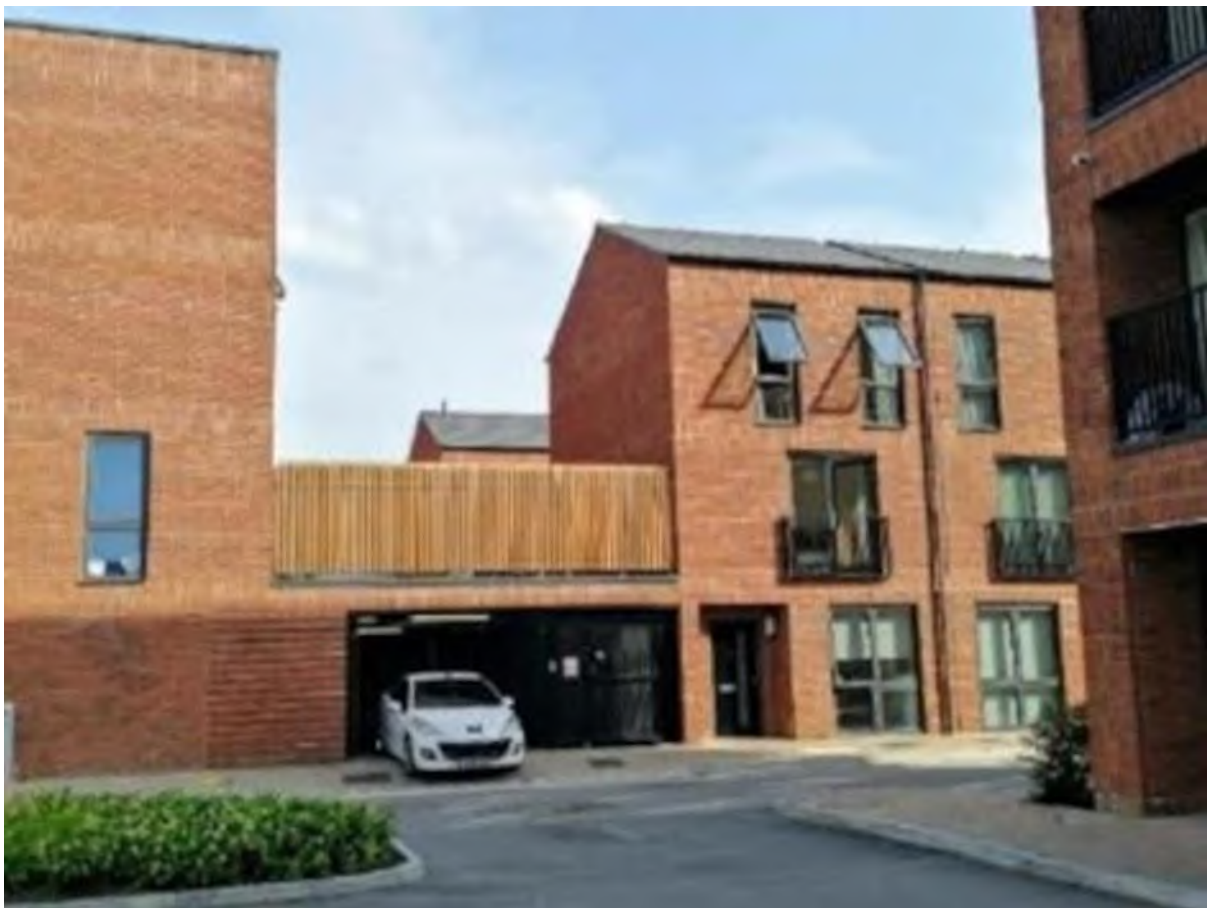
Decked 1st floor gardens over ground level parking, Greyfriars, Gloucester.
