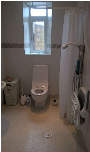
Figure 8: Adapted bathroom with level access shower and wall mounted chair
