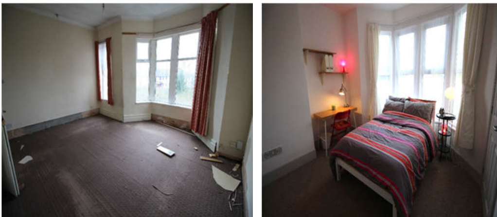
Figure 20: Front bedroom before and after refurbishment
