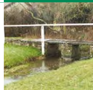
Stone footbridge - Station Road, Yate
